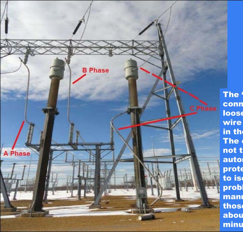
The "C" phase connection broke loose, dropping the wire to the ground in the switchyard. The open phase did not trigger automatic protection actions to isolate the problem. Operators manually took those measures about eight minutes later.
