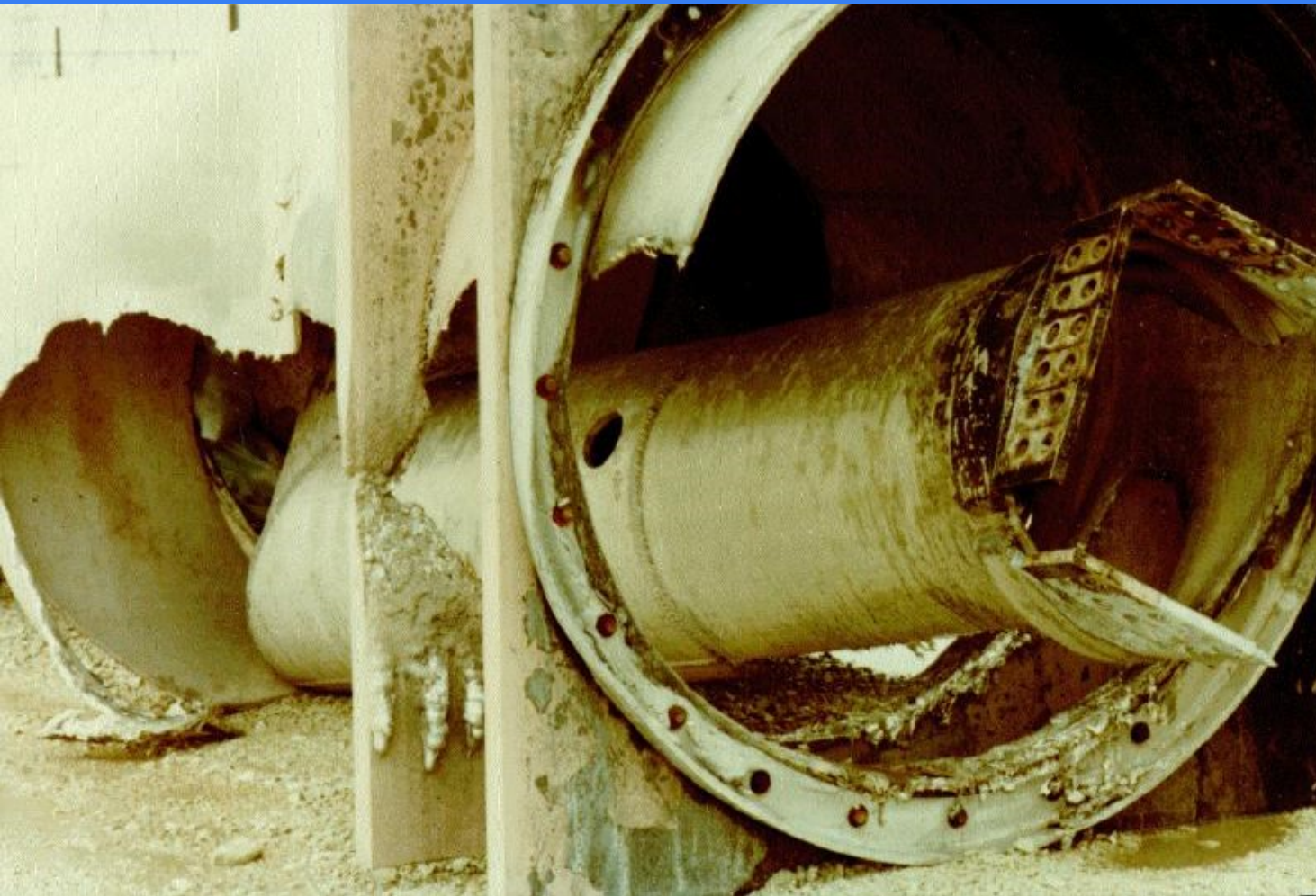
Close view of the miniflux plate area of the A-Phase bus at the transformer. Note the extensive damage to the 2" thick miniflux plate. Also note the temporary clamping ring installed after the first failure to serve as a means to attach the temporary bus duct boot.
